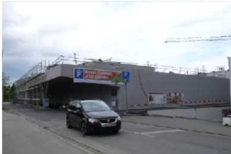
Parkhaus Migros, Oberwil
